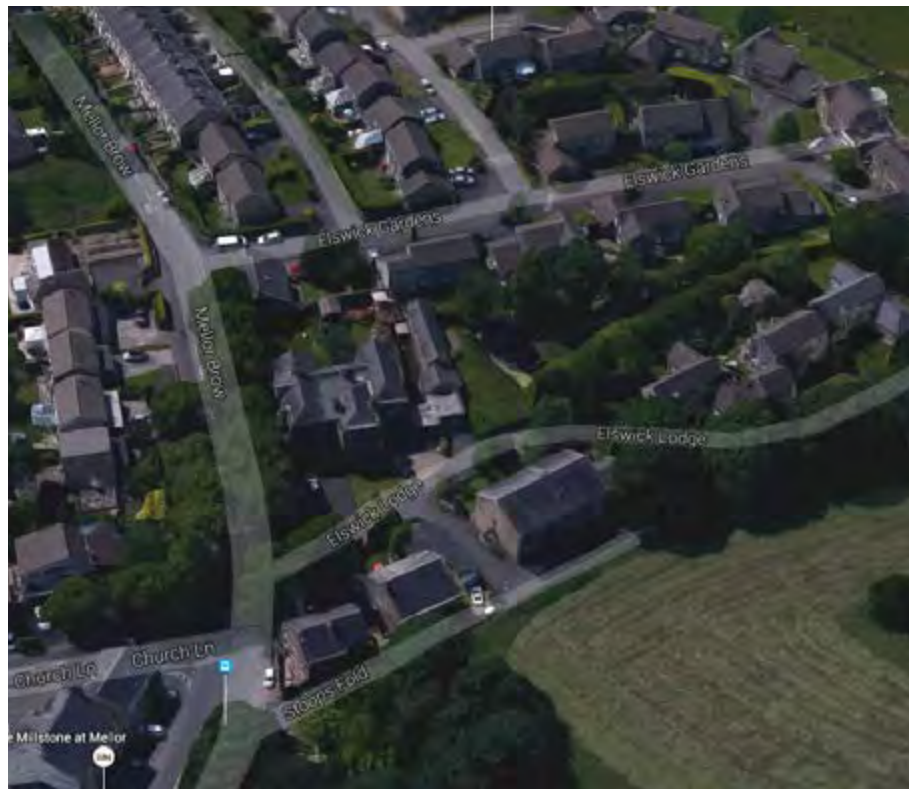
A MIX OF A FORMAL AND INFORMAL LAYOUT. THE DEVELOPMENT ALLOWS CLEAR VIEWS OF THE SURROUNDING OPEN LANDSCAPE
