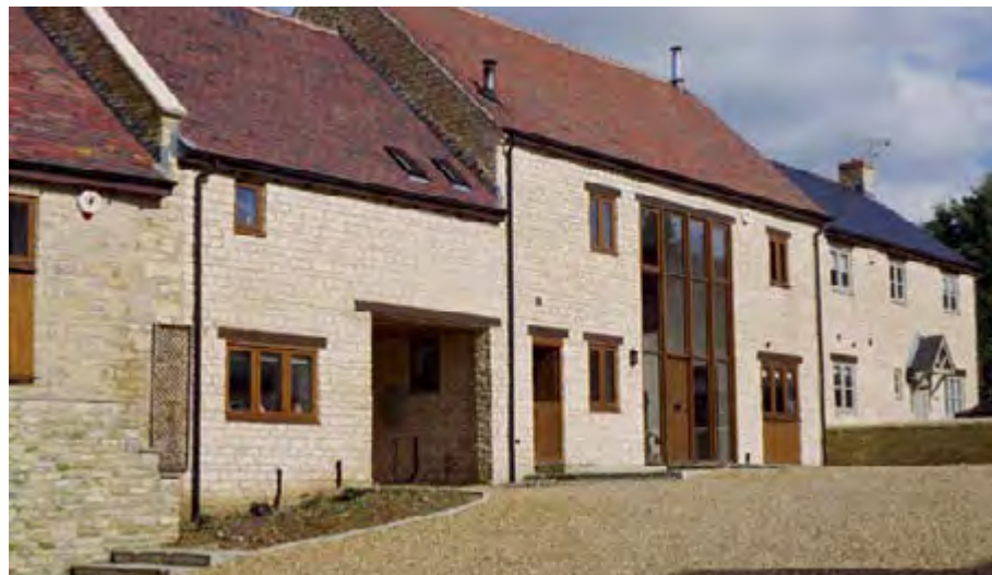
Right and far right: Traditional interpretation of Rural Typologies. Roofs step with changes in level.
