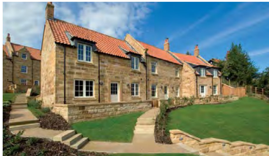
Above: Local materials such as stone is used to create a rural character within smaller terraced housing, dwellings address a green space to create a 'village character'.
